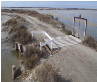
Marteliere – Wooden lock systems which allow water to circulate from one pond to another
